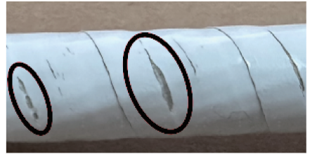
(a) 烧结裂纹
